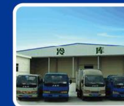
Medium temperature cold storage
